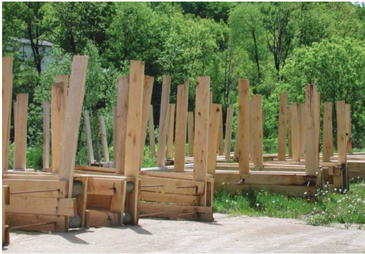
Lunkers waiting to be placed in streambanks.
