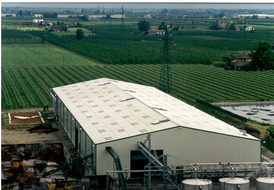
Photo 1: General view of the composting plant
