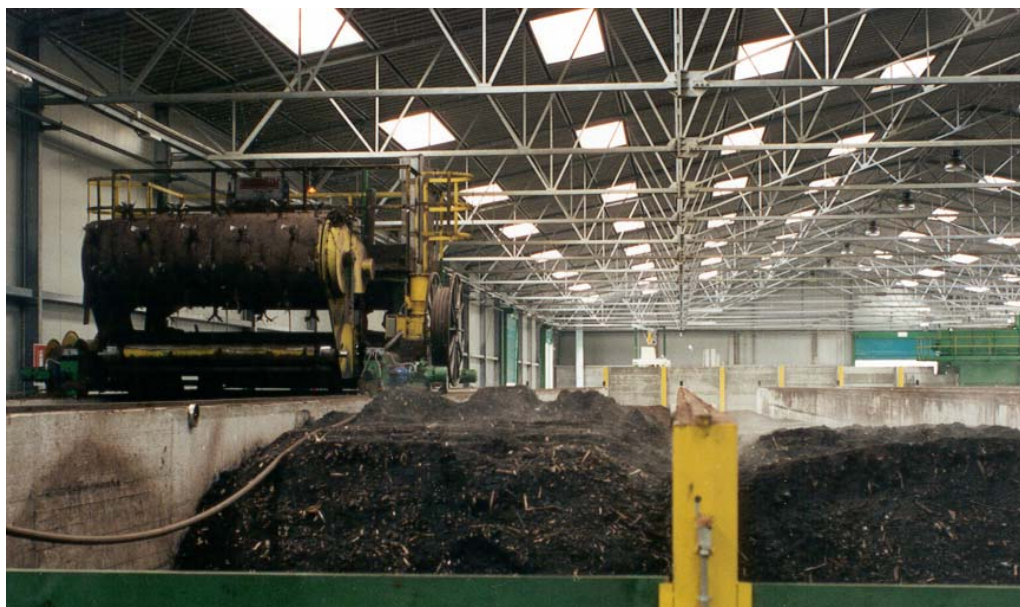
Photo 3: The mixing device during operation
